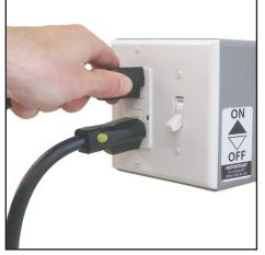
Plug the top plug (Pump Cord) back into the Power Switch located inside the sink.
