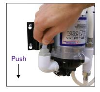
Locate Pump Inlet inside cabinet. Push Pump Inlet Quick Connect tube into white elbow fitting carefully.
